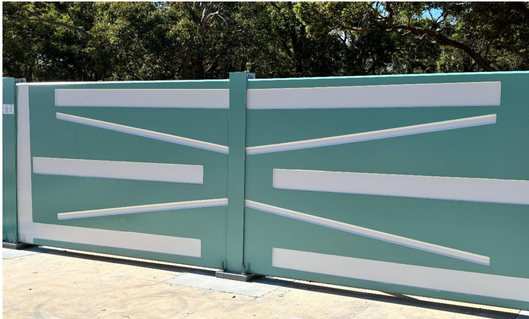
Noise panels manufactured using the JV's proprietary low carbon cement formulation which replaced 35% of traditional Portland cement with an Industrial byproduct
