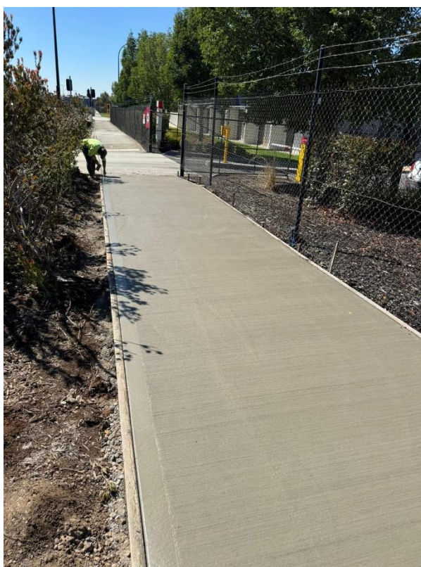
Melbourne Airport Business Park
