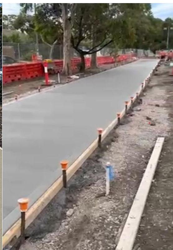
Eastern Freeway Extension Project works
