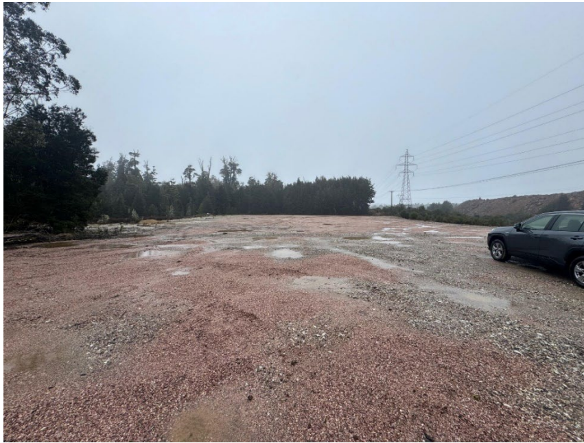
Figure 8 Graded Area on site
