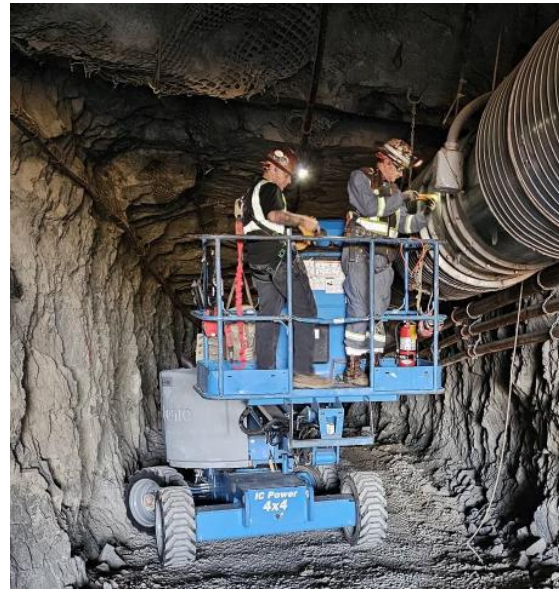
Figure 9: 4x4 articulated boom, checking ventilation fans 8 .
