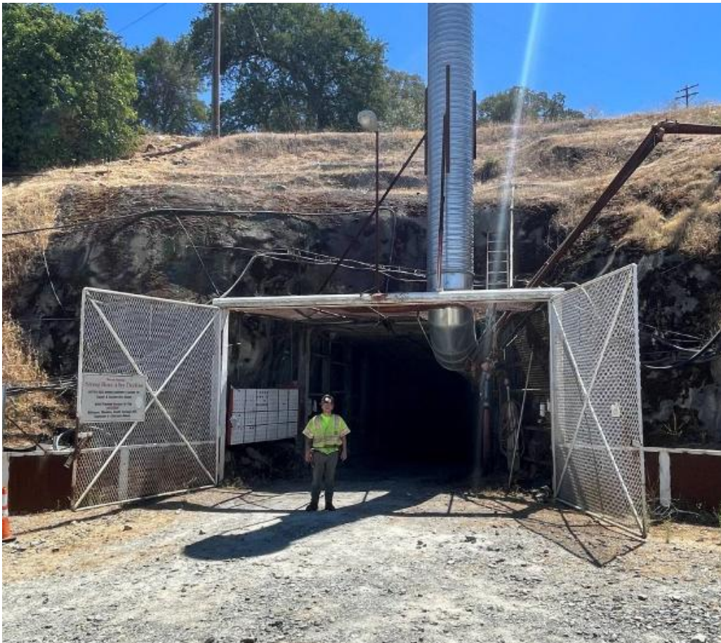
Figure 5: String Bean Alley Decline unlocked and open for action. The Decline is nearly 900m long, at a decline of 12%, attaining a depth of around 200m below surface.
