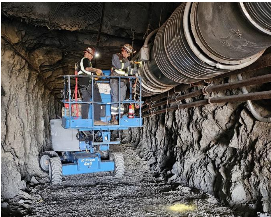
Figure 8: Recently purchased 4x4 articulated boom performing checks on ventilation fan at Stringbean Alley Decline portal. The work platform provides a stable platform as the Company advances pumping equipment and drops ventilation at the water interface.
