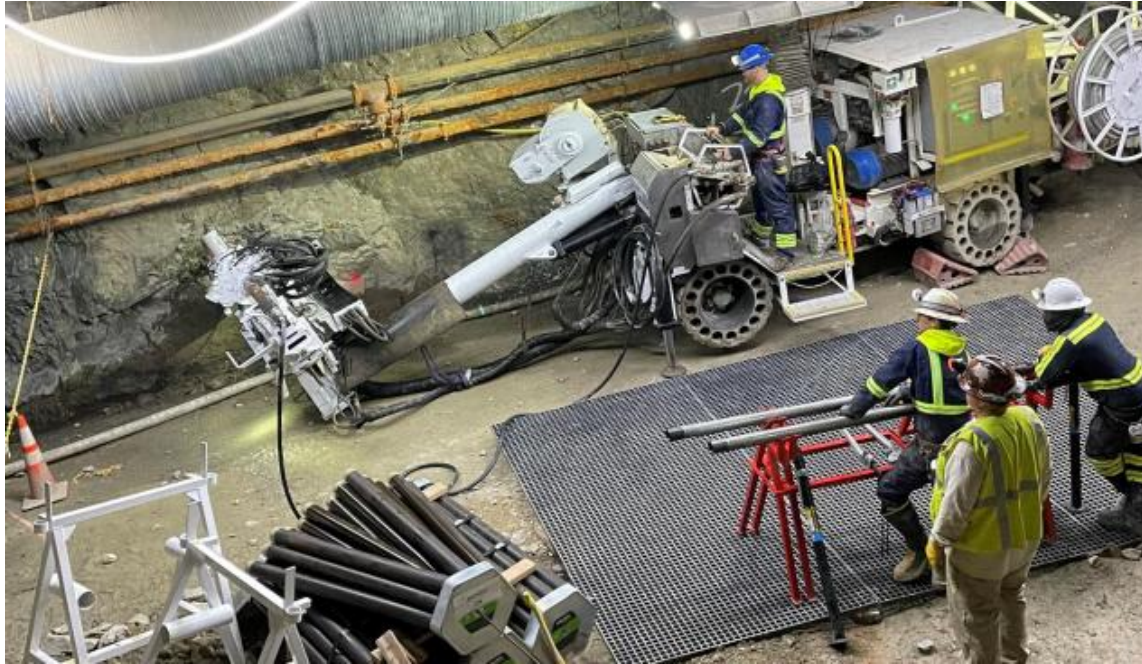
Figure 10: Swick Gen II underground diamond drill rig, drilling DDH251 at crosscut 3 (XC3).
