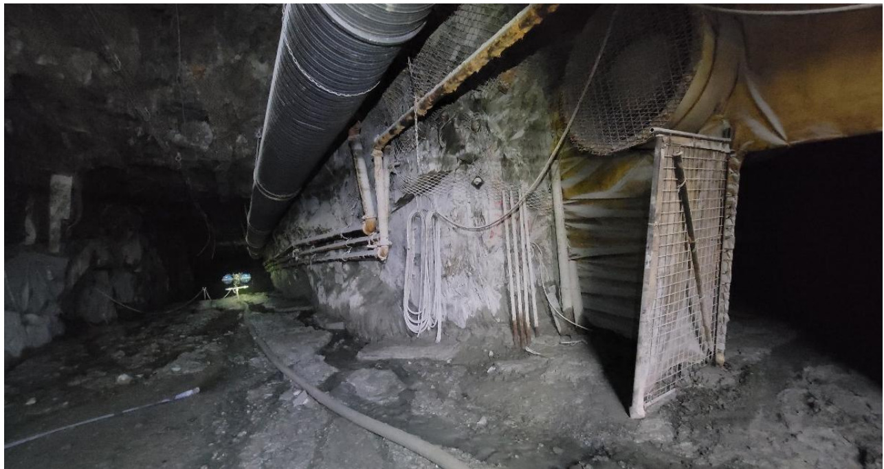
Figure 6: Dewatering continuing below XC8.
