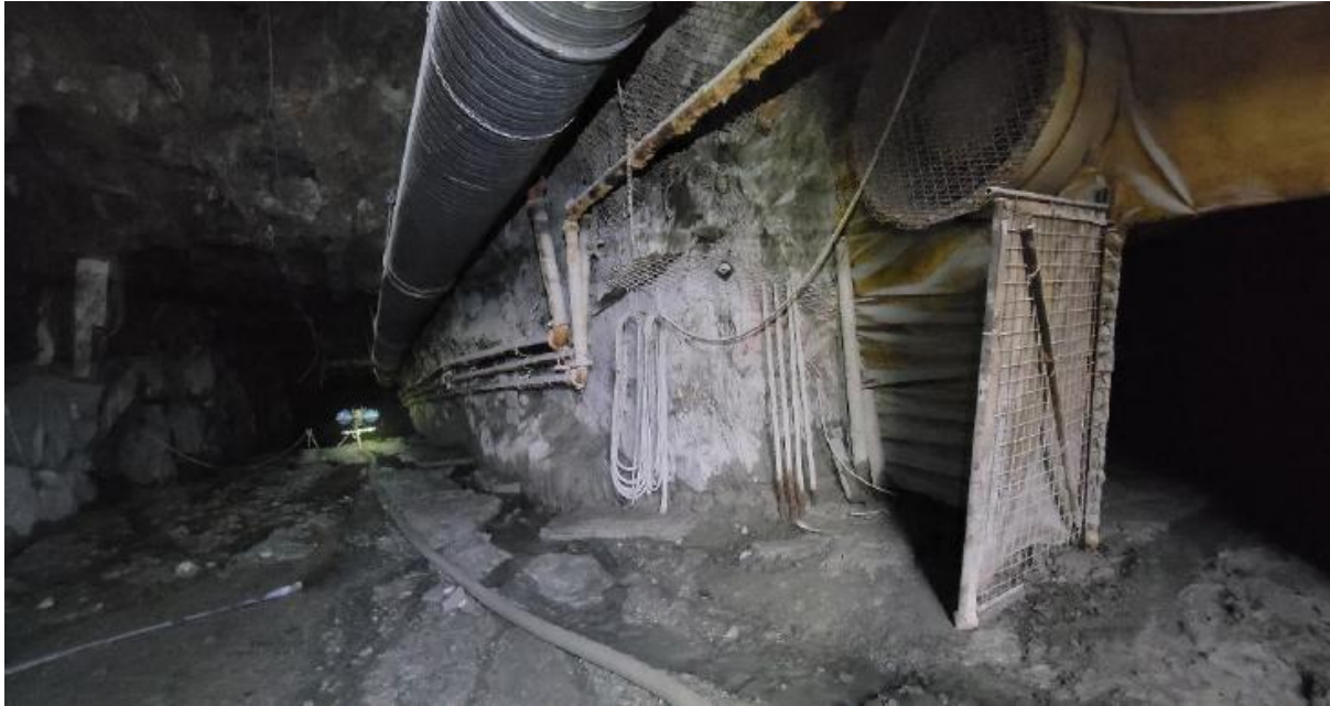
Figure 12: Dewatering continuing below XC8 7
