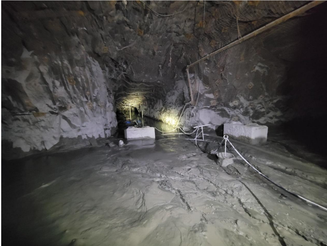
Figures 1a&b: Pumping activities below XC11 immediately in front of decline sump, Stringbean Alley Decline (Wednesday am 5 th August PST).
