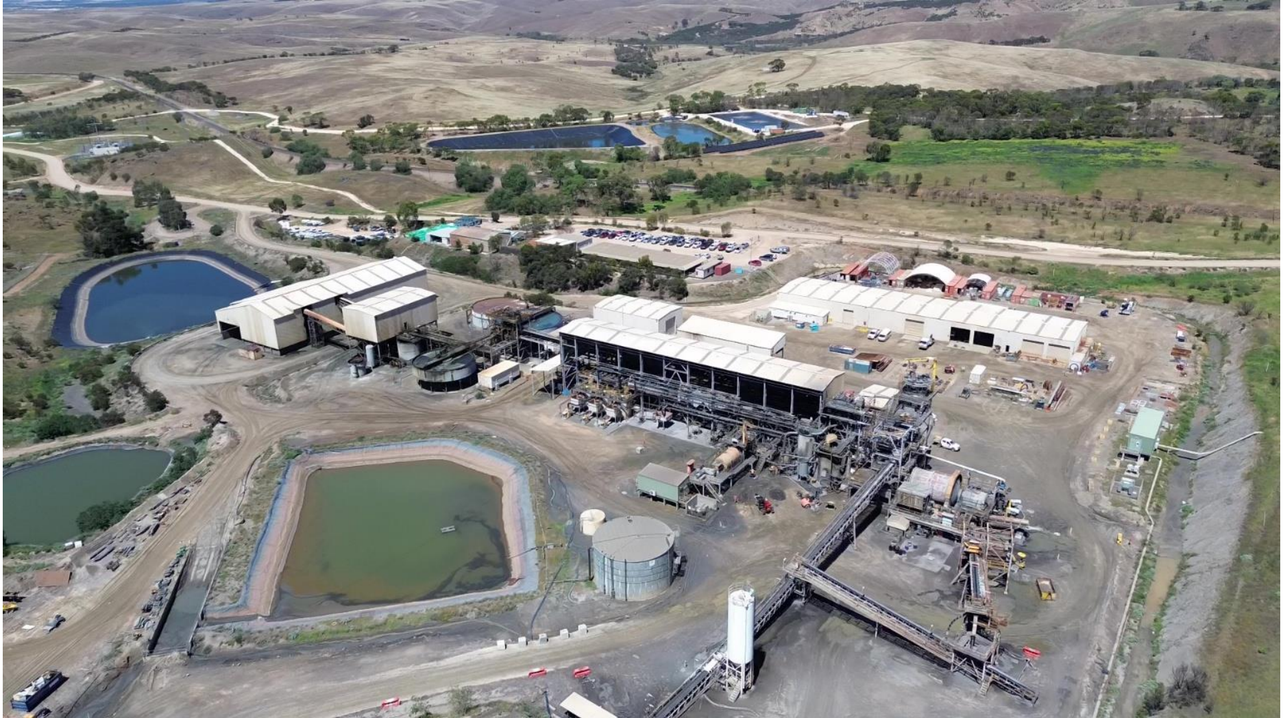
Figure 2 – Kanmantoo Copper Gold Mine Processing Plant
