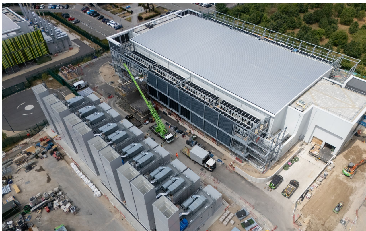
Construction underway at Kao’s KLON-03 facility
