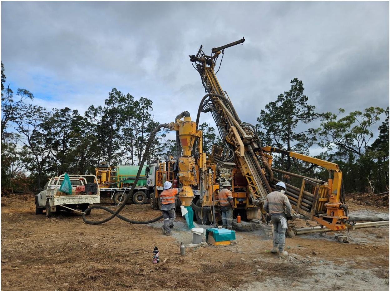
Figure 2 Drill Rig No. 2 (wheel mounted RC rig) drilling at the Orient Silver-Indium Project
