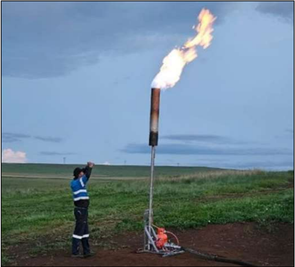
Figure 3 – Gas flaring from well 271-06PT
