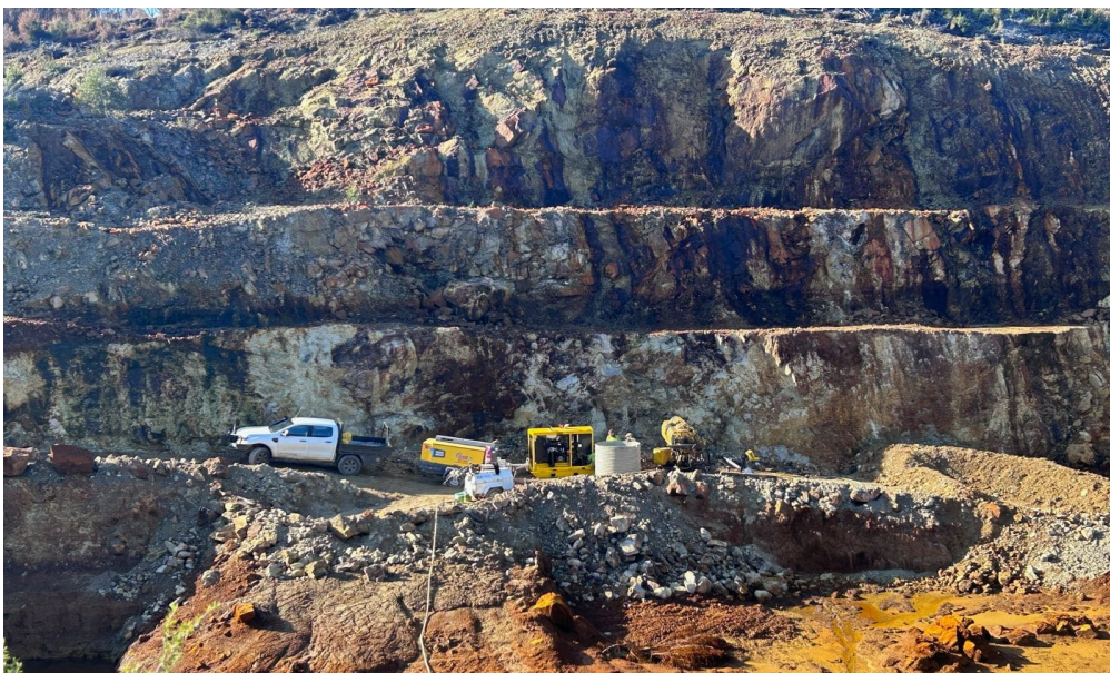
Figure 9 Granville East pit
