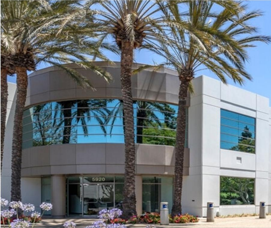
NEW LUMOS FACILITY · CARLSBAD, CALIFORNIA
