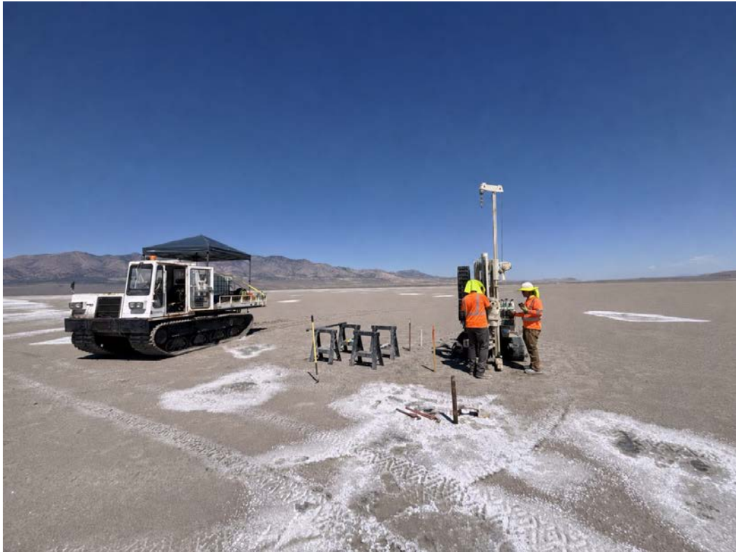
Figure 15: Drilling of Upper Aquifer using a Direct Push Rig at White Plains Lithium Brine Project
