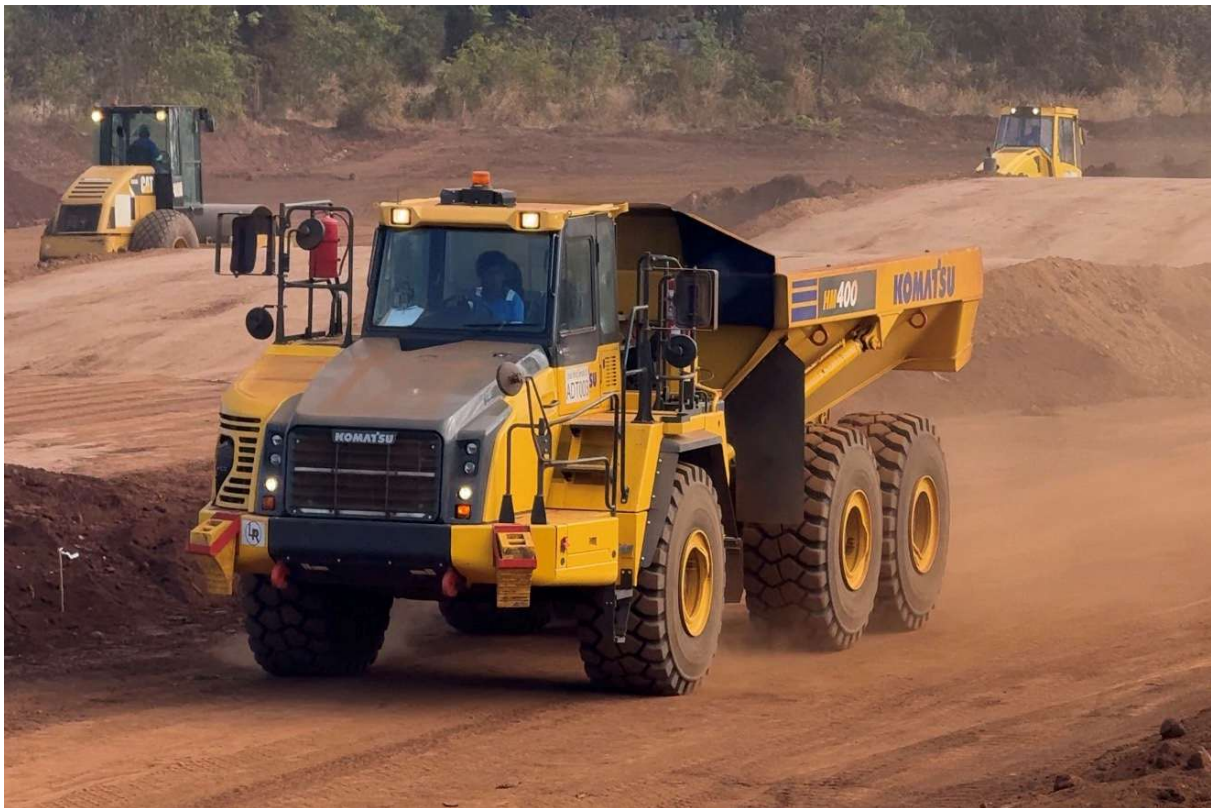
Picture 6. Civil works continuing in the Tailings Storage Facility
