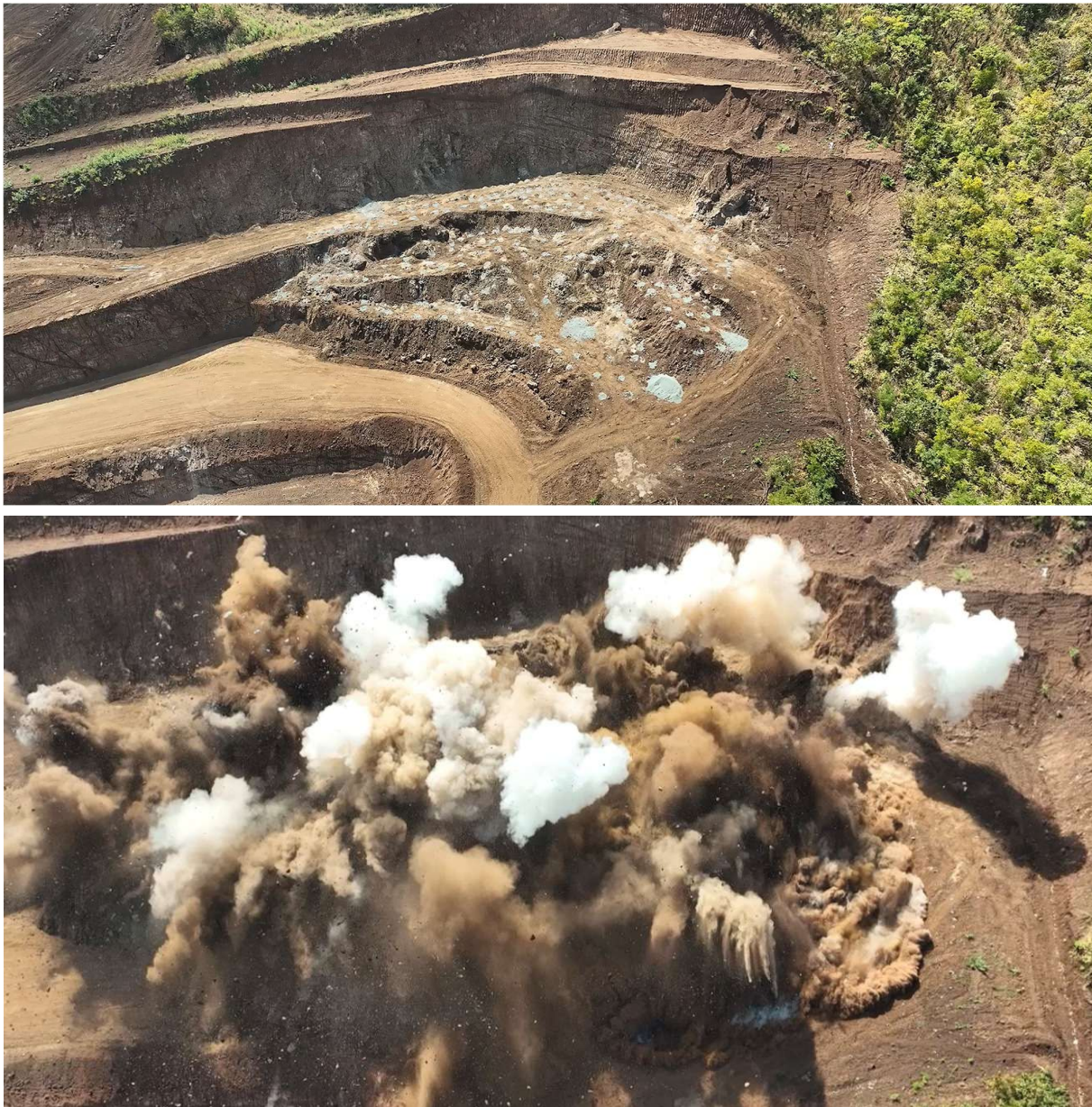
Picture 1. Aerial views of the drill pattern and first blast
