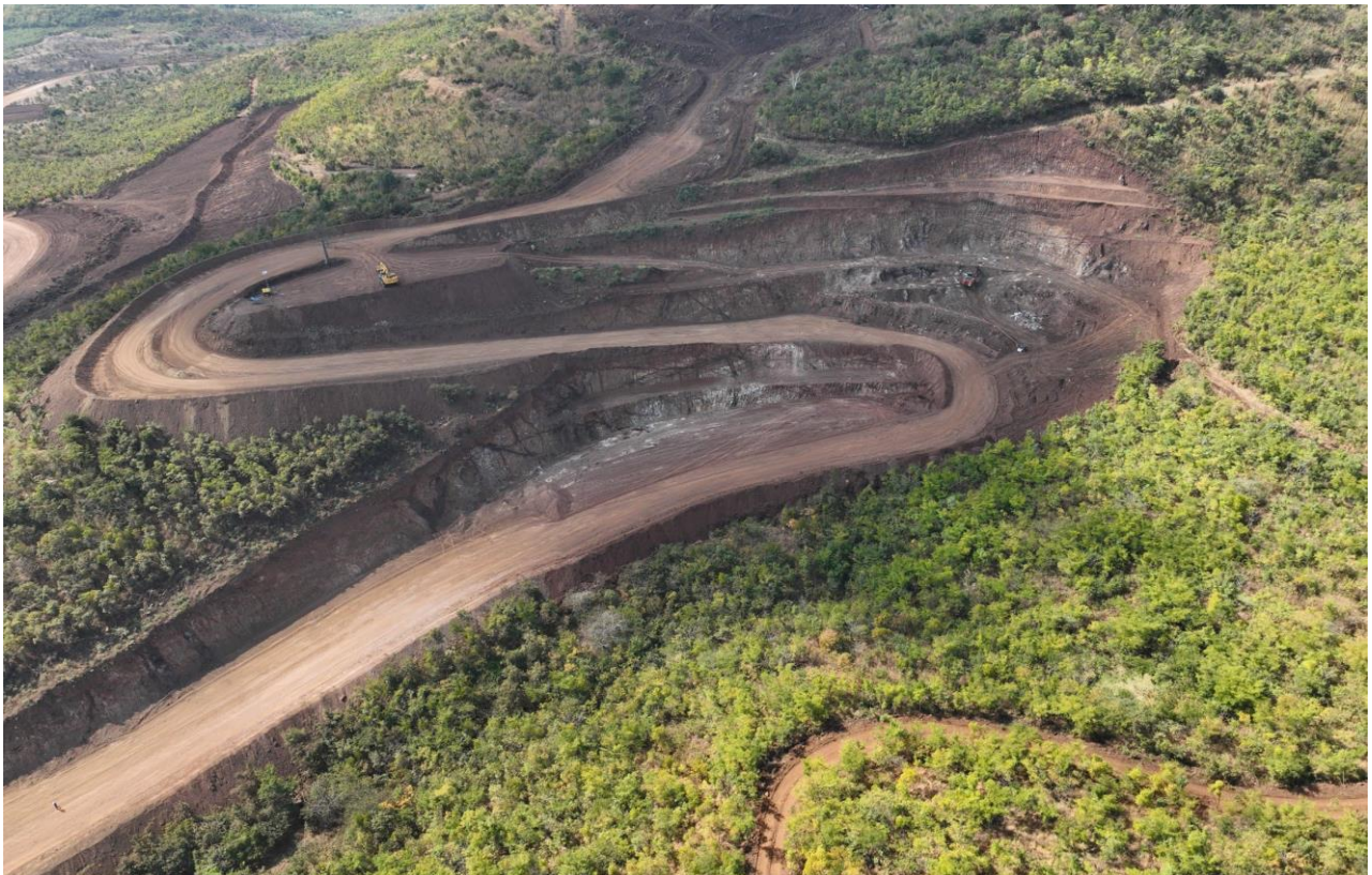
Picture 4. Completed haul road providing access to the Stage 1 pit area
