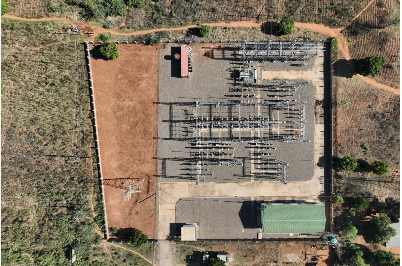
Picture 10. Balaka ESCOM substation tie-in point for the power corridor
