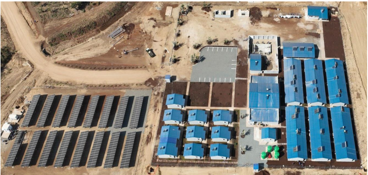
Picture 12. Kangankunde Timpe 90-personnel accommodation camp.
