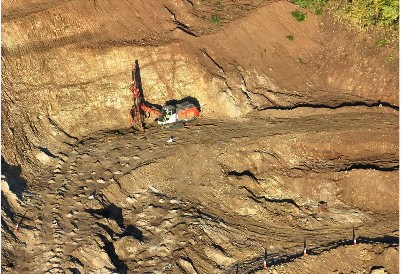
Picture 3. Production drill rig drilling the first blast pattern at the Stage 1 pit area, marking a key mining readiness milestone ahead of the planned first blast at Kangankunde
