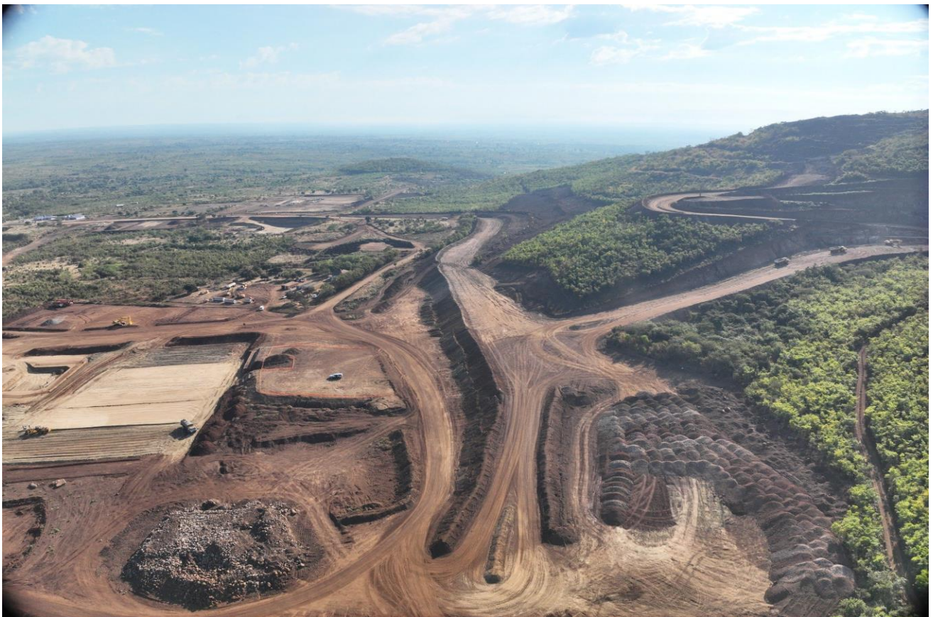
Picture 6. ROM pad and mining skyway
