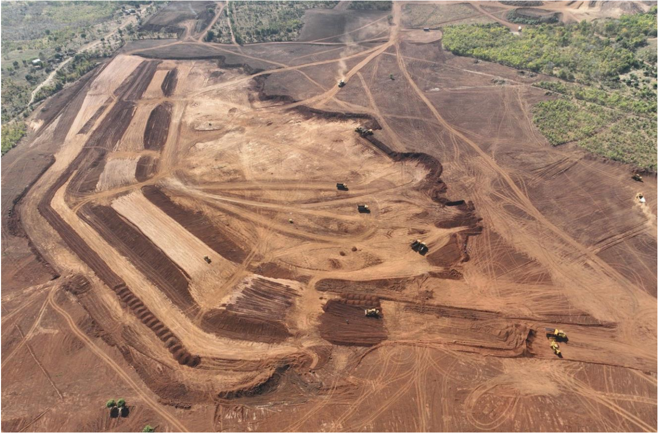
Picture 8. Kangankunde Tailings Storage Facility Progress
