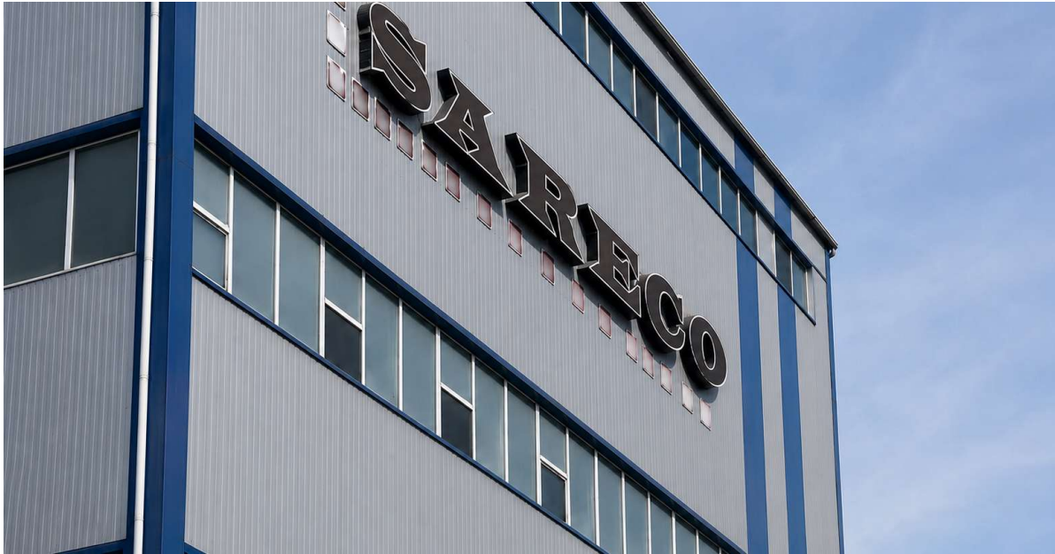
Picture 3. Operating SARECO MREC facility in Stepnogorsk, Kazakhstan.
