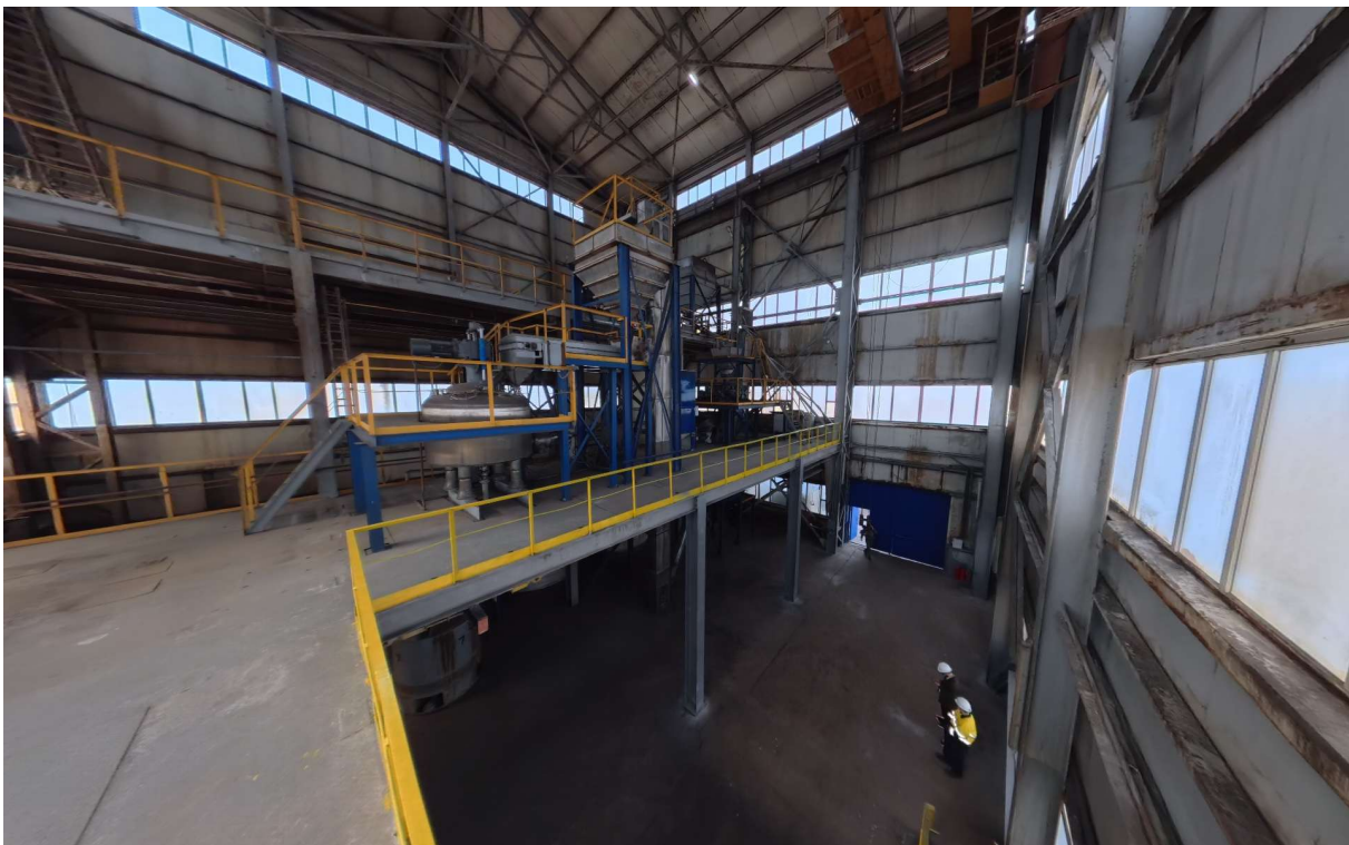
Picture 9. Additional images of the existing infrastructure at the SARECO MREC Facility.
