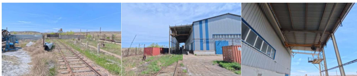
Picture 6. Rail siding and rail car unloading infrastructure at the SARECO Facility
