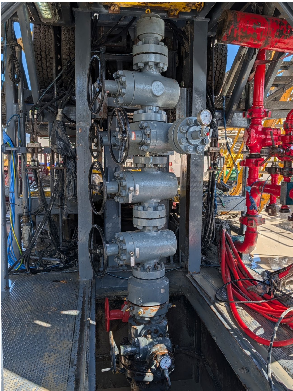
Figure 1 Completed well head
