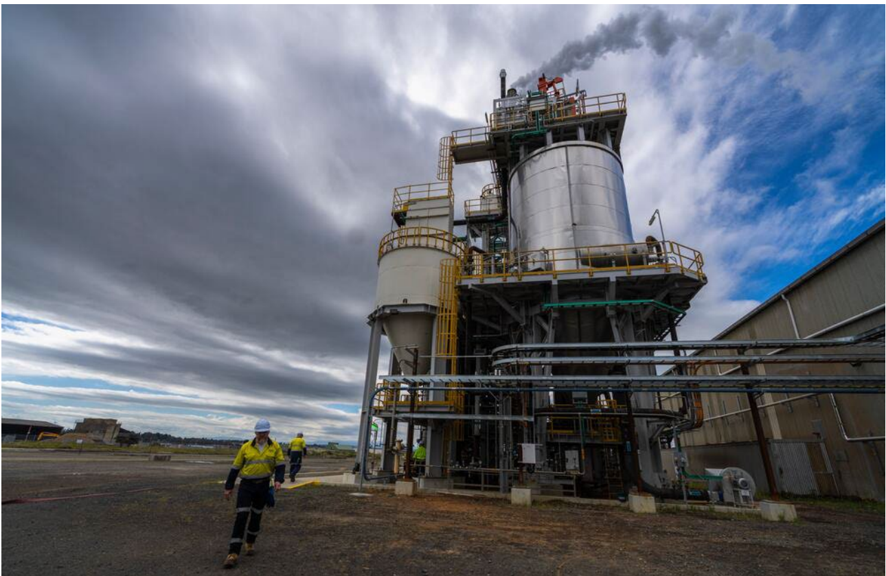
Spray Roaster operations resumed post repair of fan defect.
