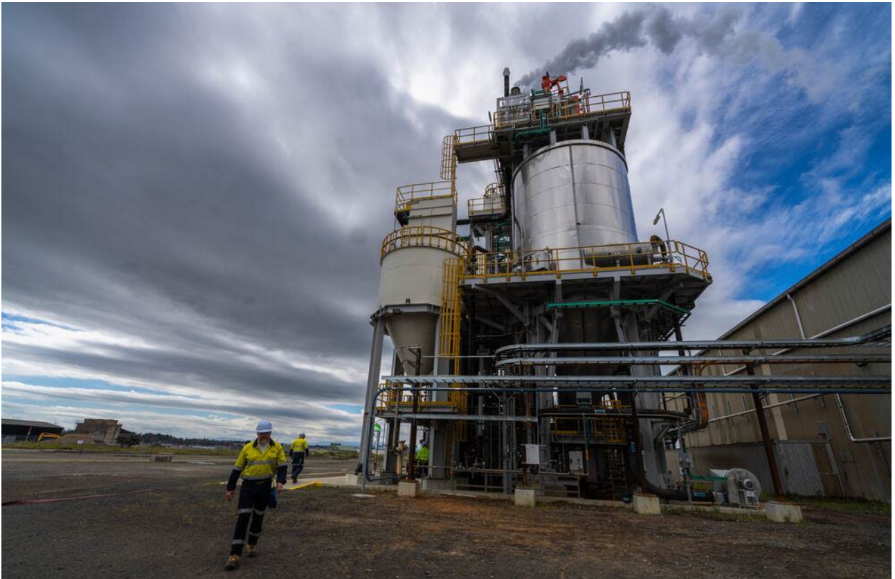
Figure: Spray Roaster operations resumed post repair of fan defect.
