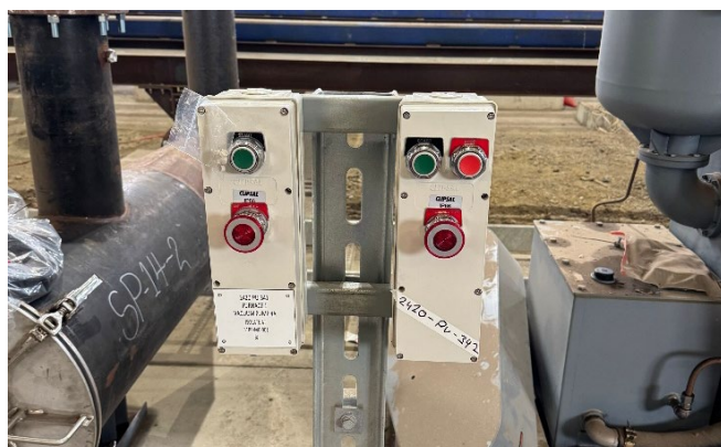
Reduction Furnace local junction boxes & main panel installation complete
