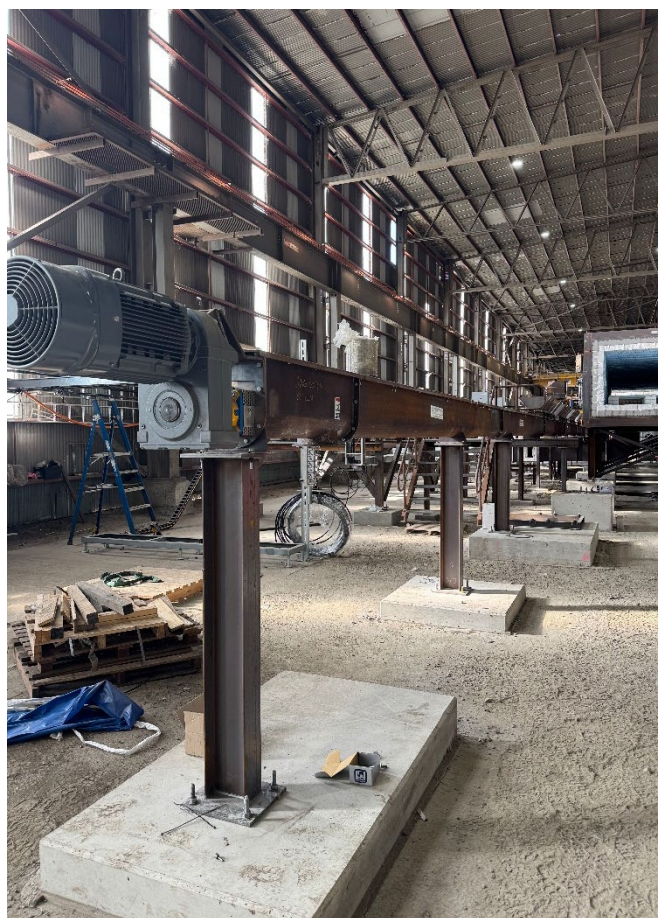
Quicklime piping and Reduction Furnace screw conveyor and platform installation complete
