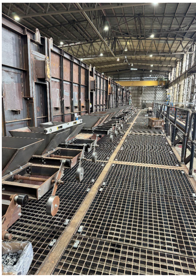
Quicklime piping and Reduction Furnace screw conveyor and platform installation complete
