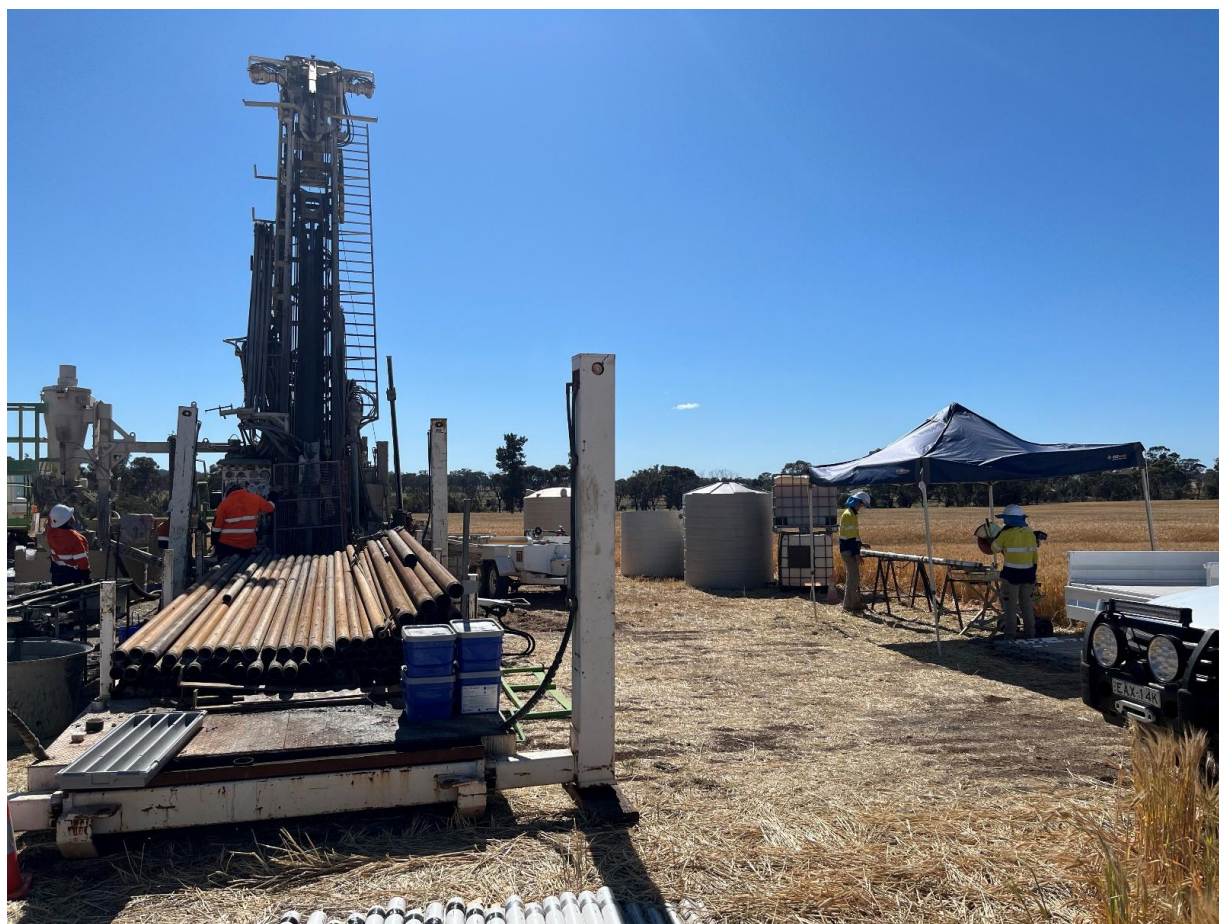
Figure 5: Drill Rig mobilised at the Dam deposit.
