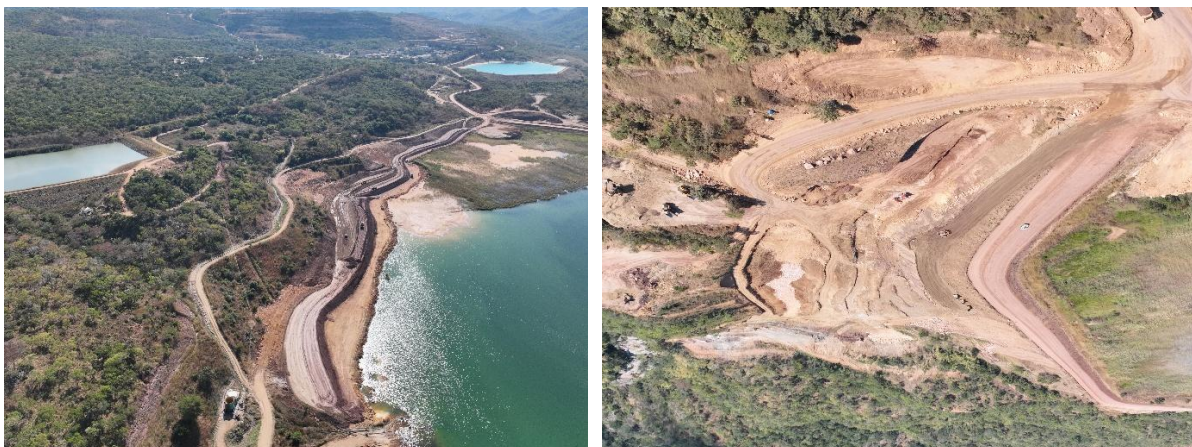
Figures 3 and 4: TSF expansion works, June 2026
