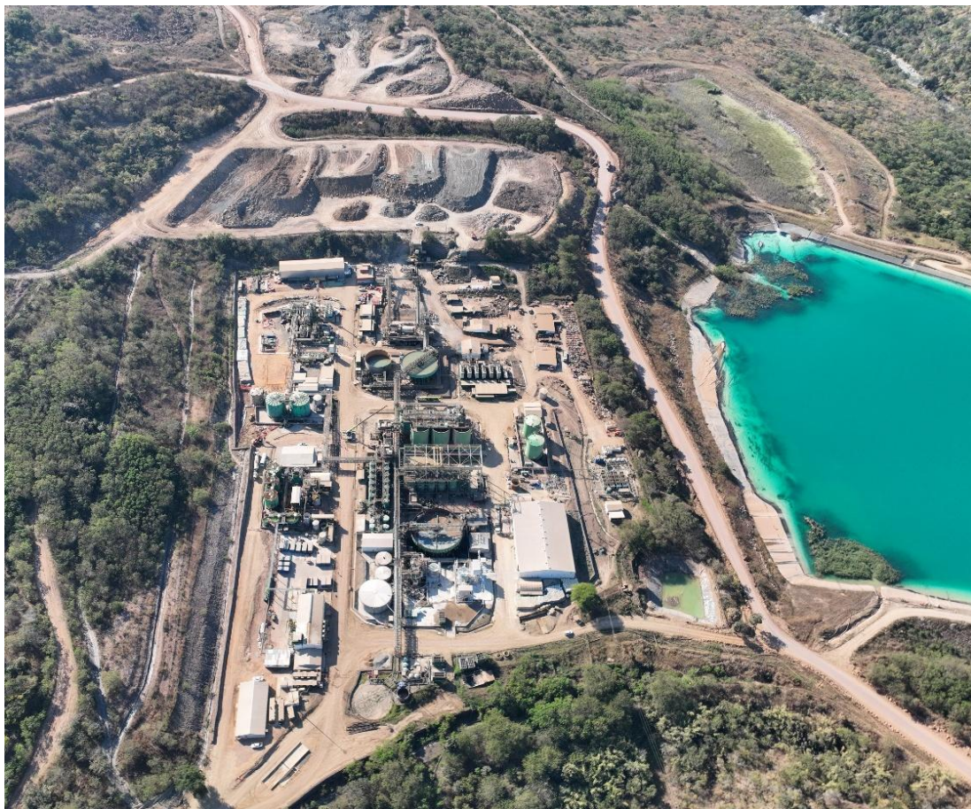
Figure 1: Kayelekera processing plant and ROM stockpile area, June 2026.
