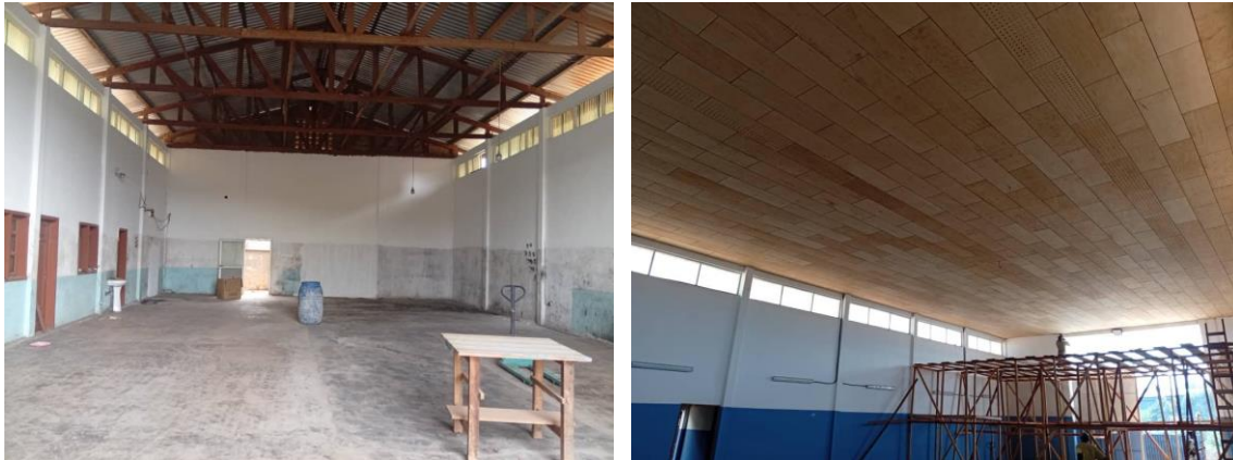
Figure 3: Photos of the LRM Yaoundé laboratory under construction and retrofit.
