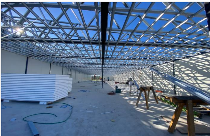
Progress at permanent Mine Services Area (MSA)
