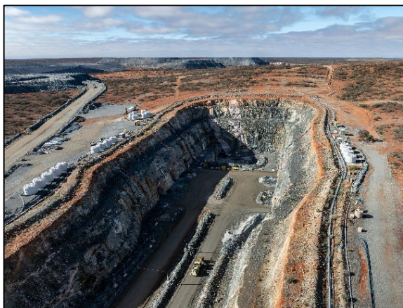
Figure 7: Infrastructure preparation at North-West Flats
