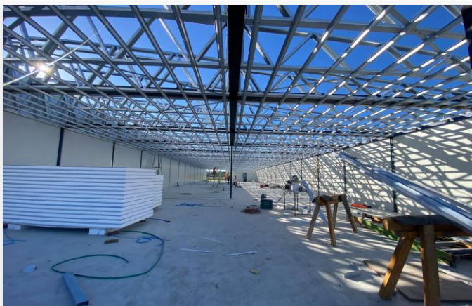
Progress at permanent Mine Services Area (MSA)
