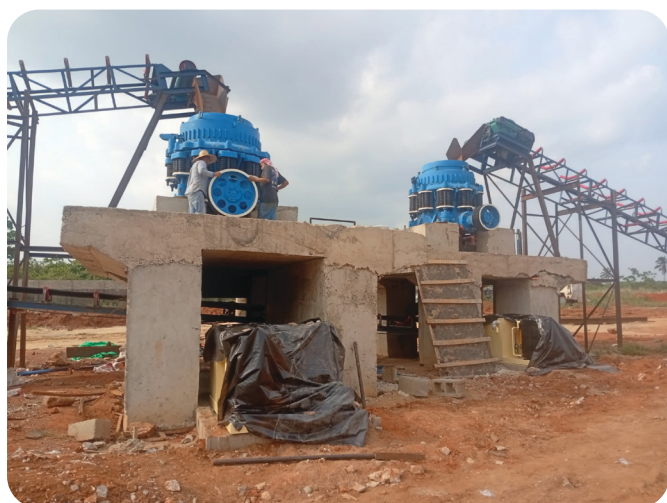
Figure 3. Construction underway on the spodumene concentrator in north-west Nigeria
