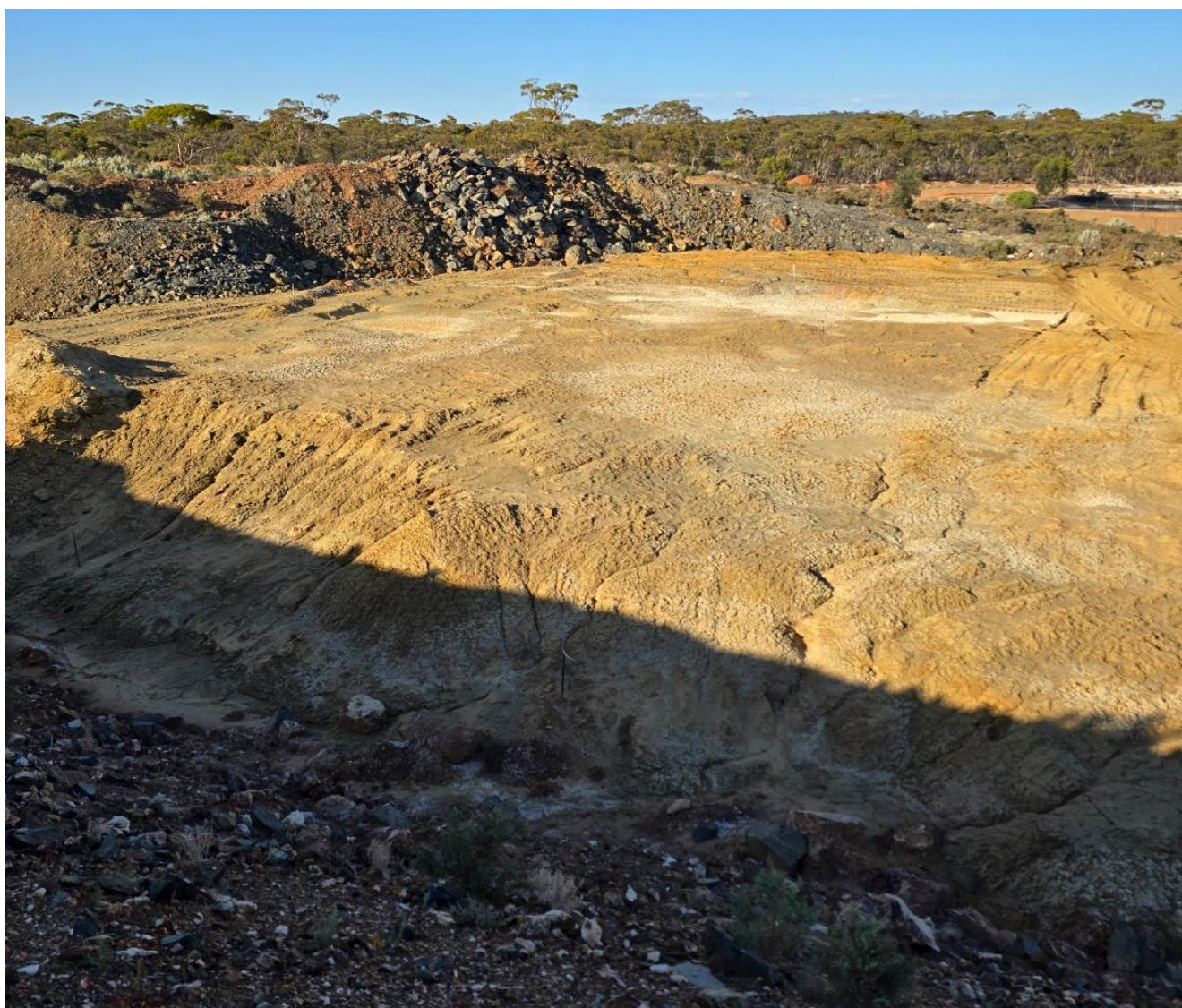
Figure 3: SW Tailings Dam
