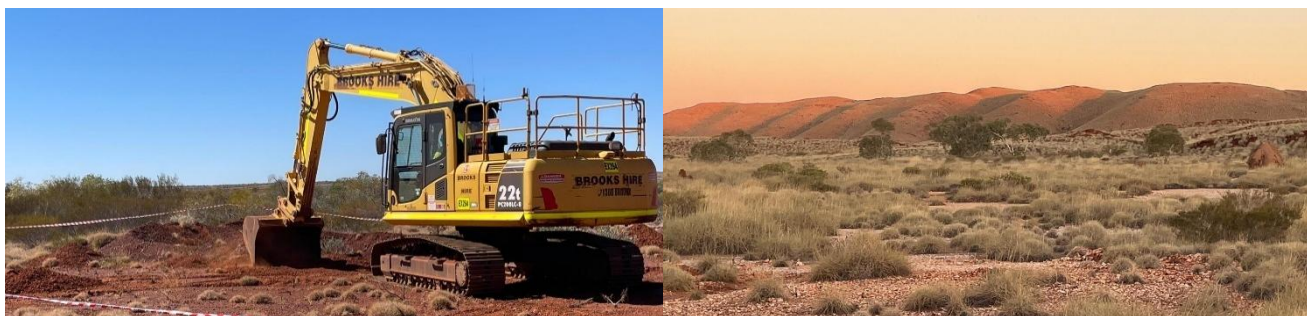
Figure 6 - Macro Mining Services performing works onsite at South Woodie Woodie in July 2026 (post reporting period).
