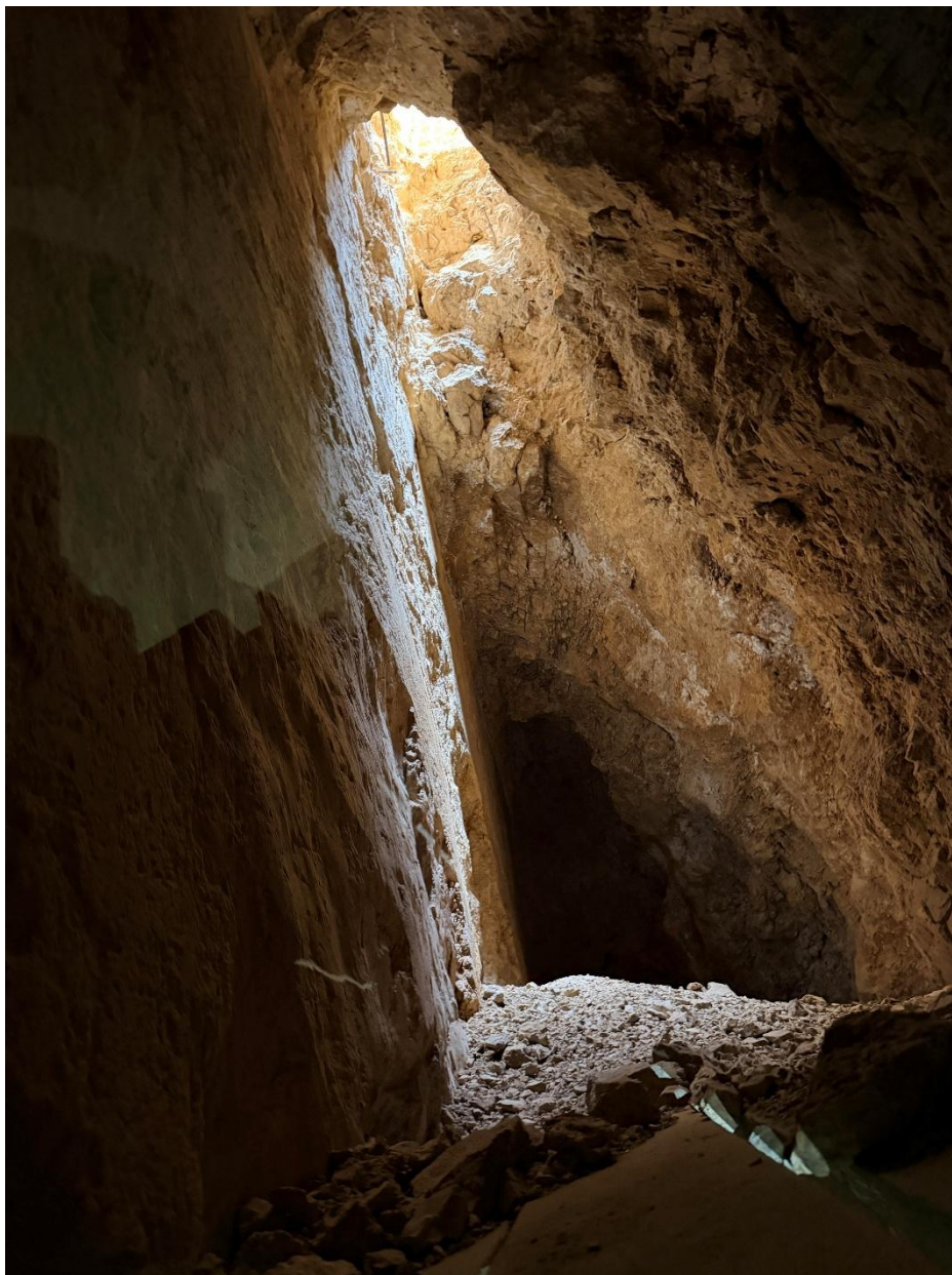
Figure 1: Blue Dick Underground Stope daylighting to surface
