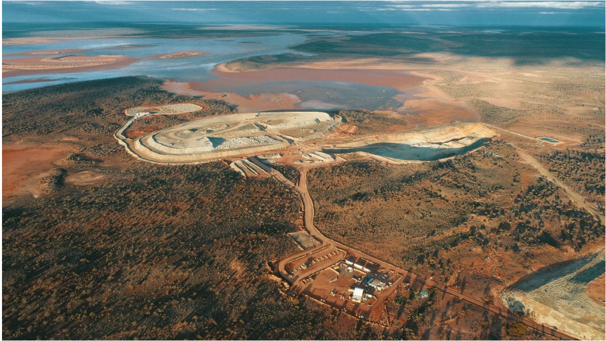
Plate 2: Oblique view of the Devon operation looking east with offices and maintenance workshop in the foreground – note flooding at Lake Carey in the background after heavy rains
