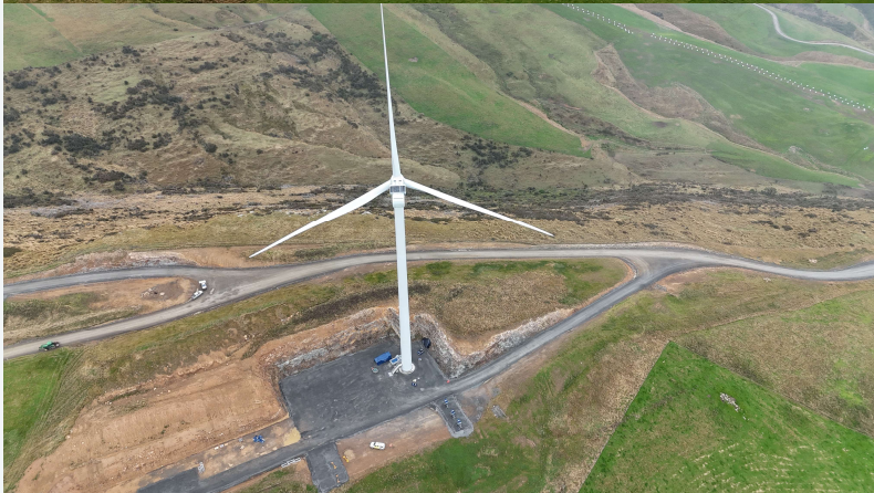
Kaiwera Downs Stage 2 under construction
