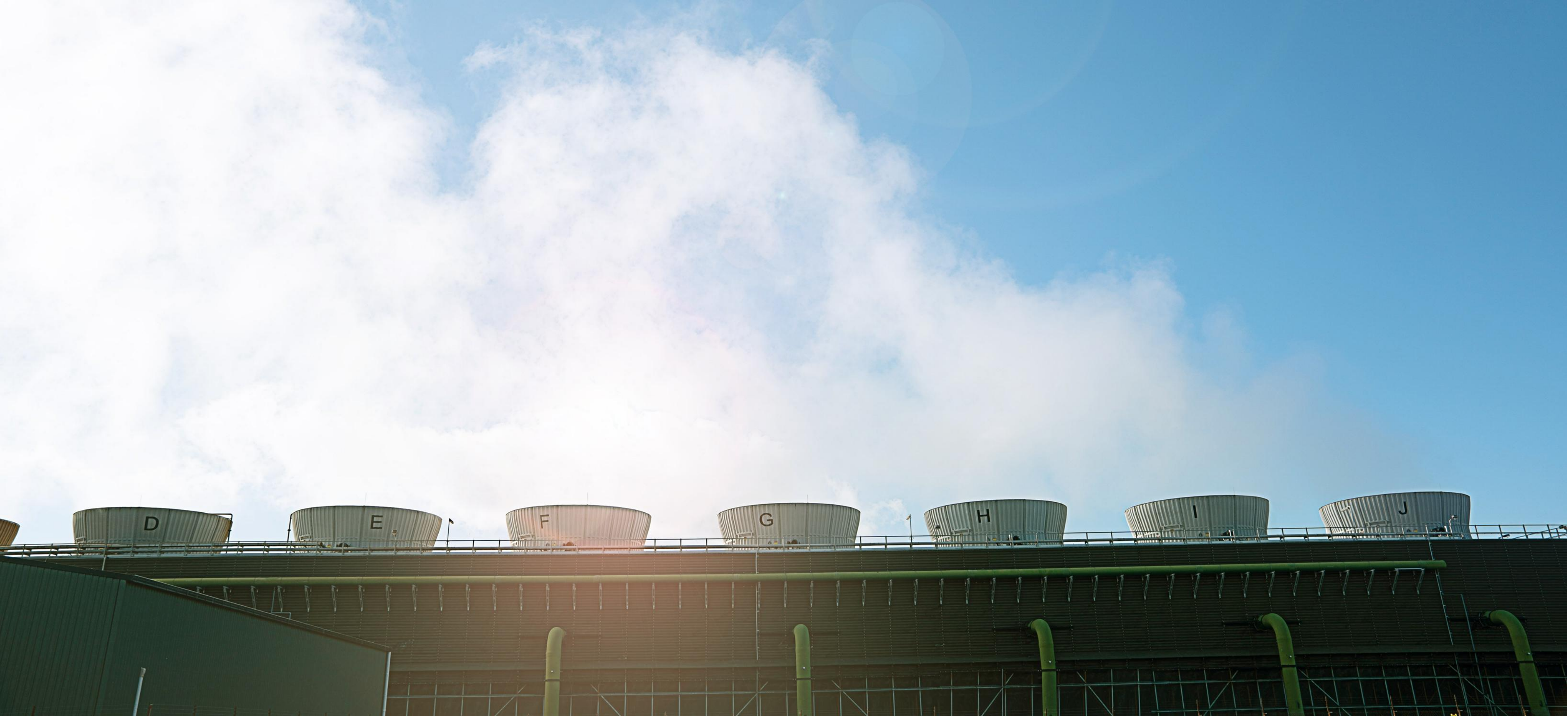
Ngā Awa Pūrua cooling tower
