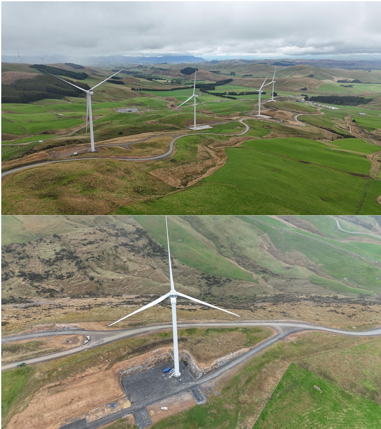
Kaiwera Downs Stage 2 under construction
