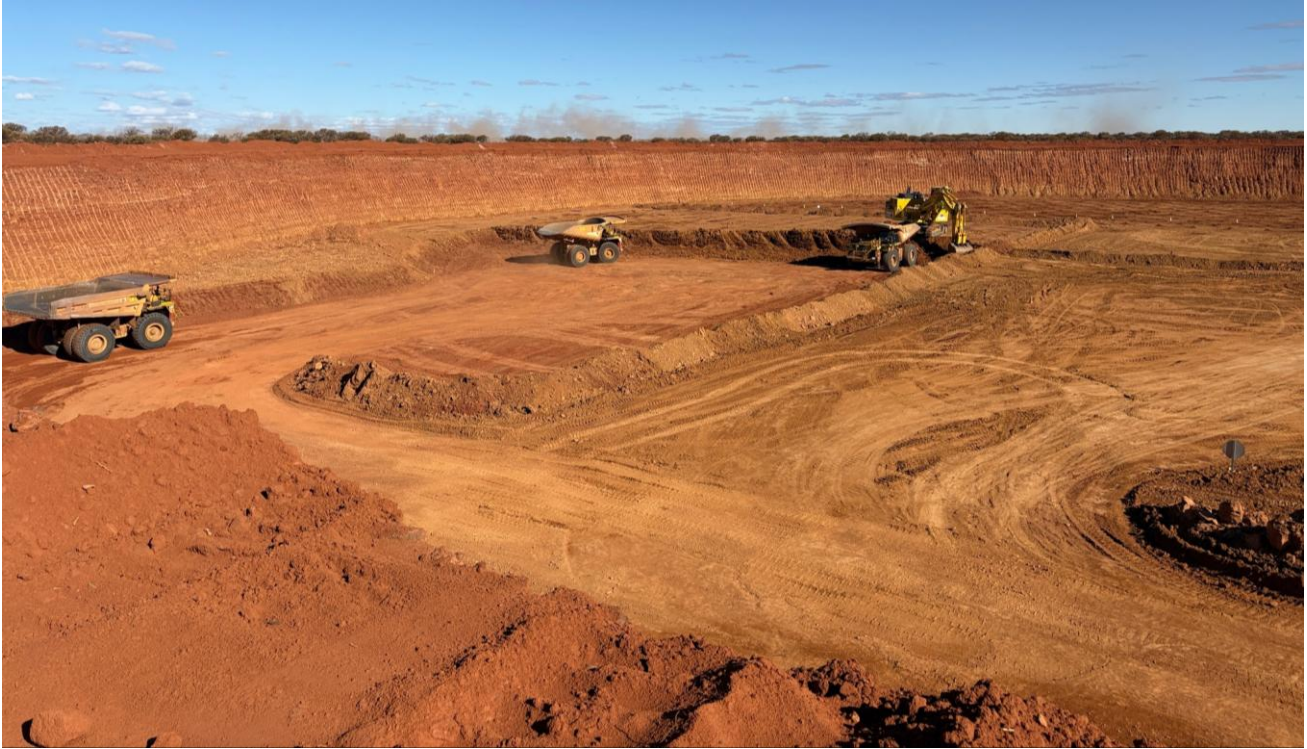
Figure 1: Stripping Stage 1 Turnberry South open pit.
