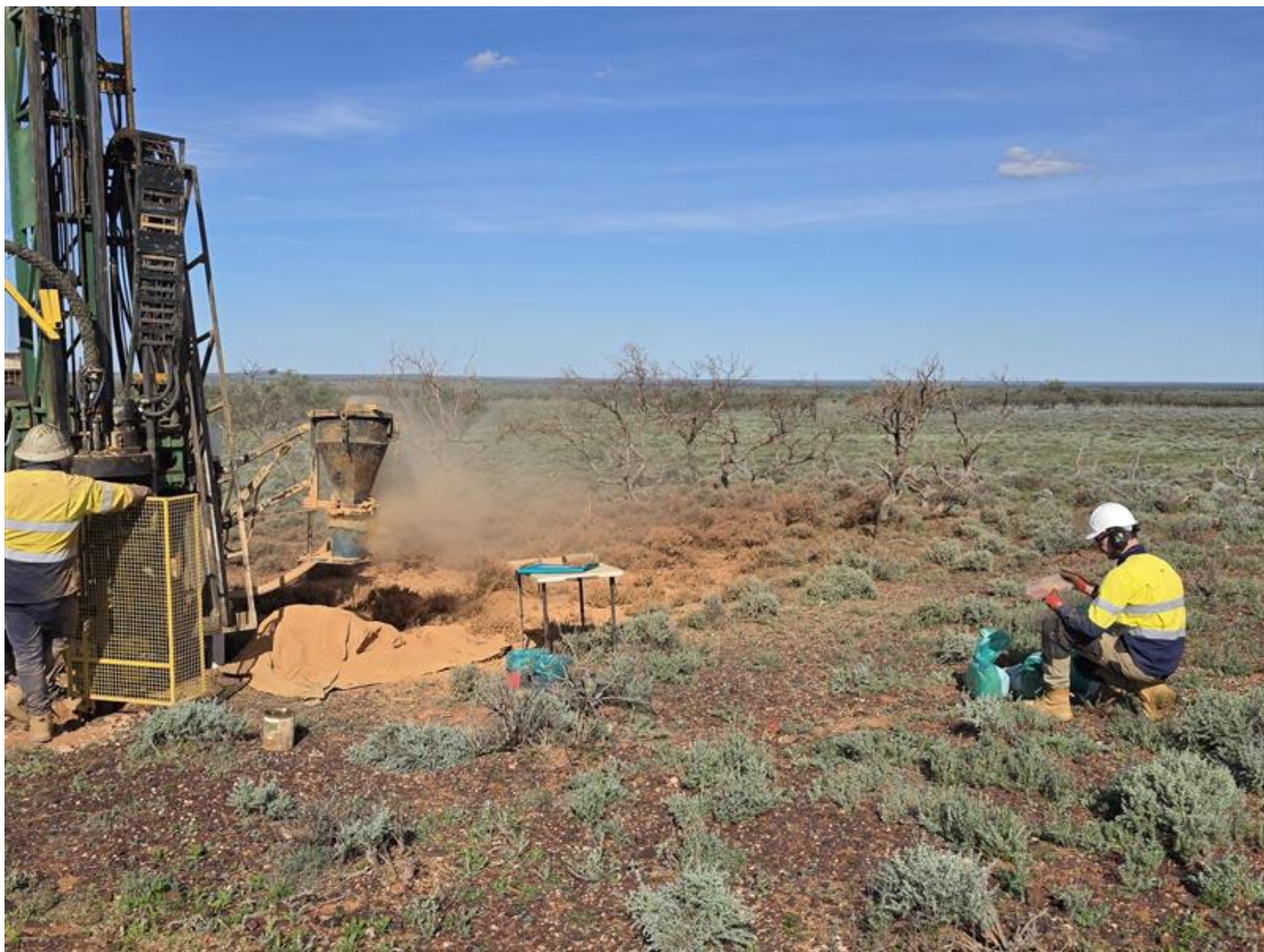
Figure 2. Air core drill rig, drilling at the Ironback Hill REE Prospect
