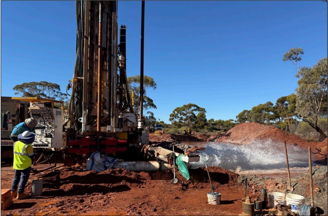
Figure 4: Water bore airlift testing and installation
