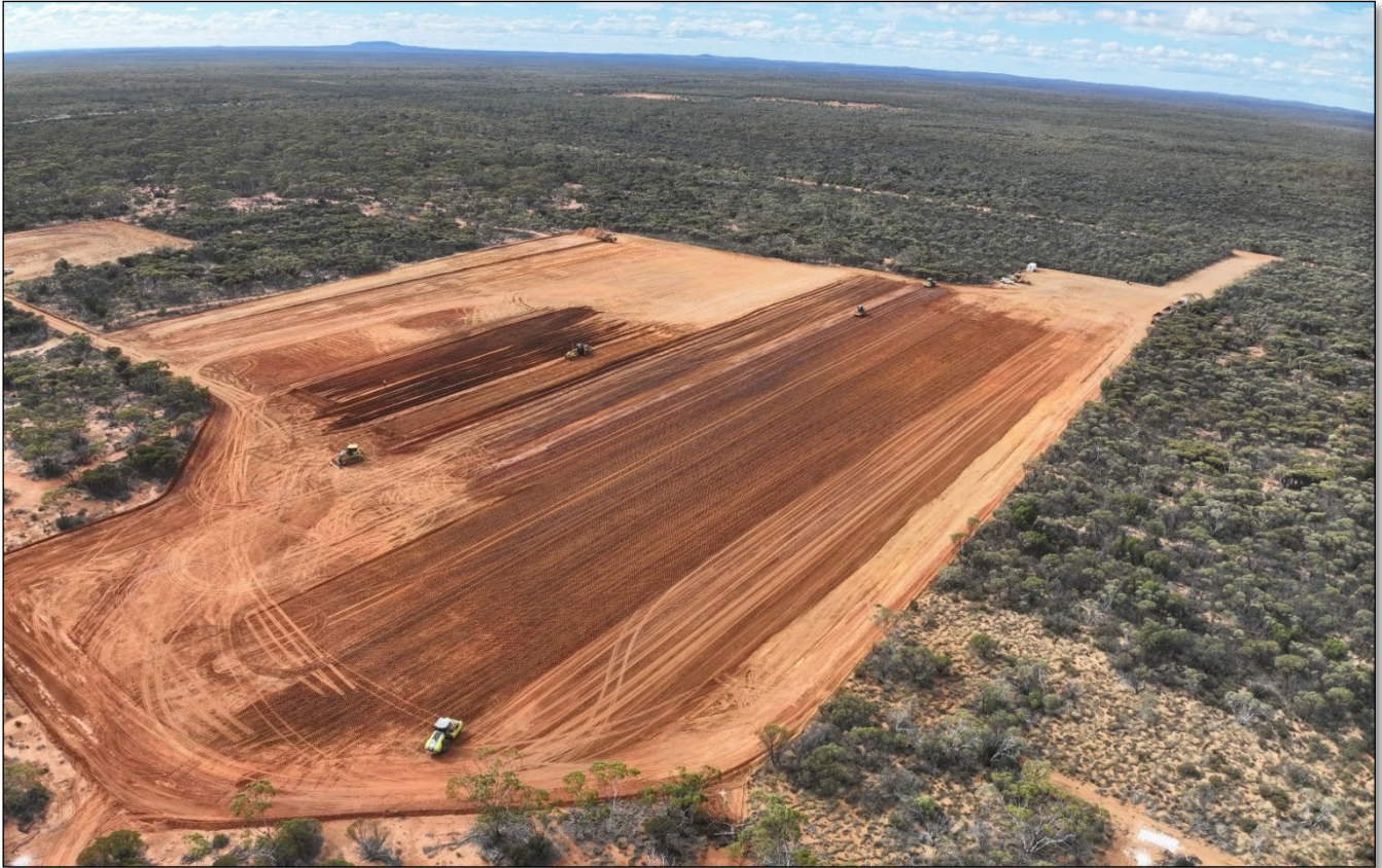
Figure 2: Bulk earthworks for the accommodation village
