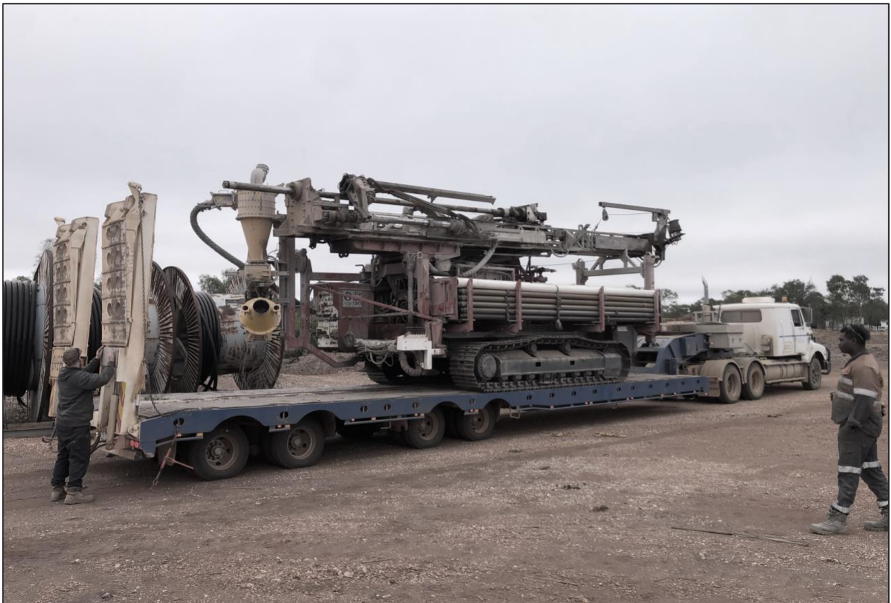
Figure 1: Eagle Drilling RC Rig arriving at location of the Peak Downs Copper Prospect
