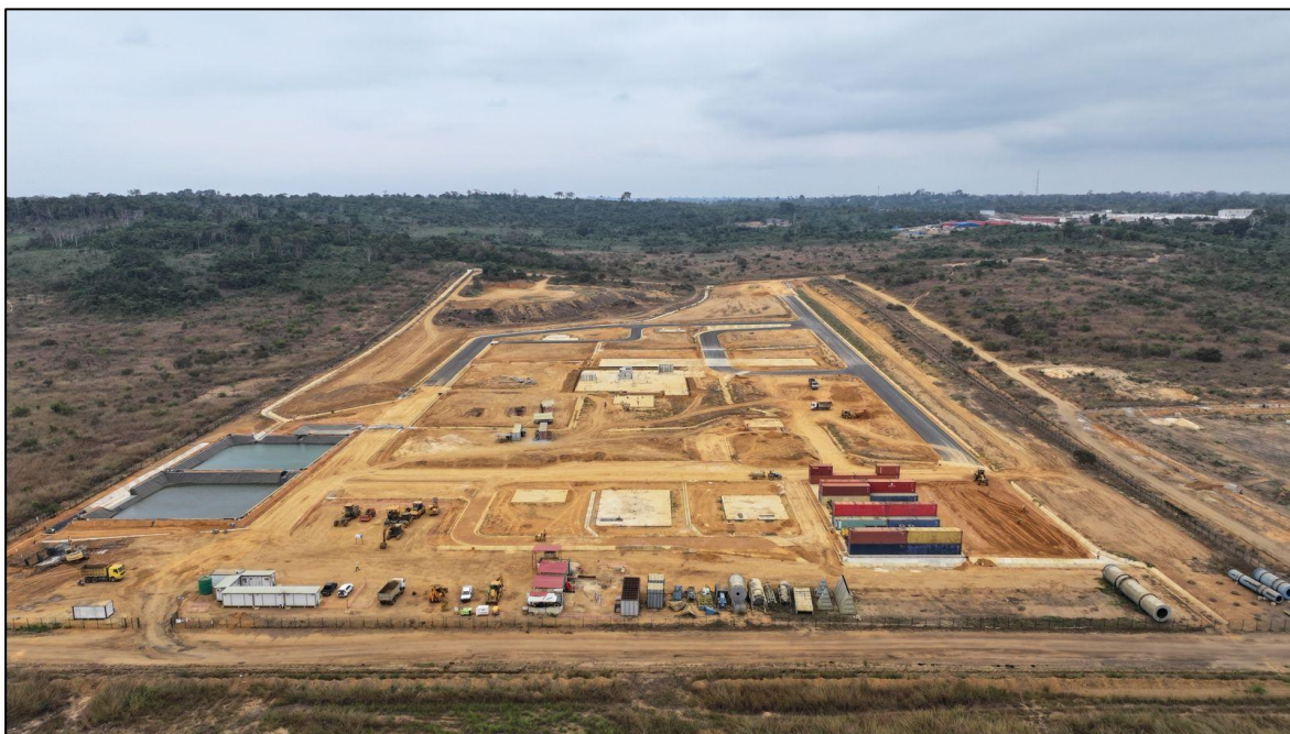
Figure 1 – Construction progress from the Cabinda Phosphate Fertilizer Plant, located in Cabinda, Angola.
