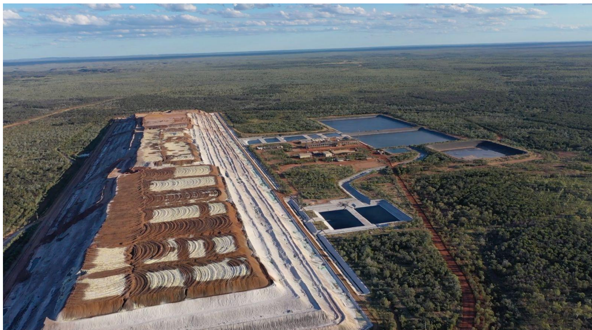
Figure 3: Aerial view of Austral's Mt Kelly Copper Processing Facility
