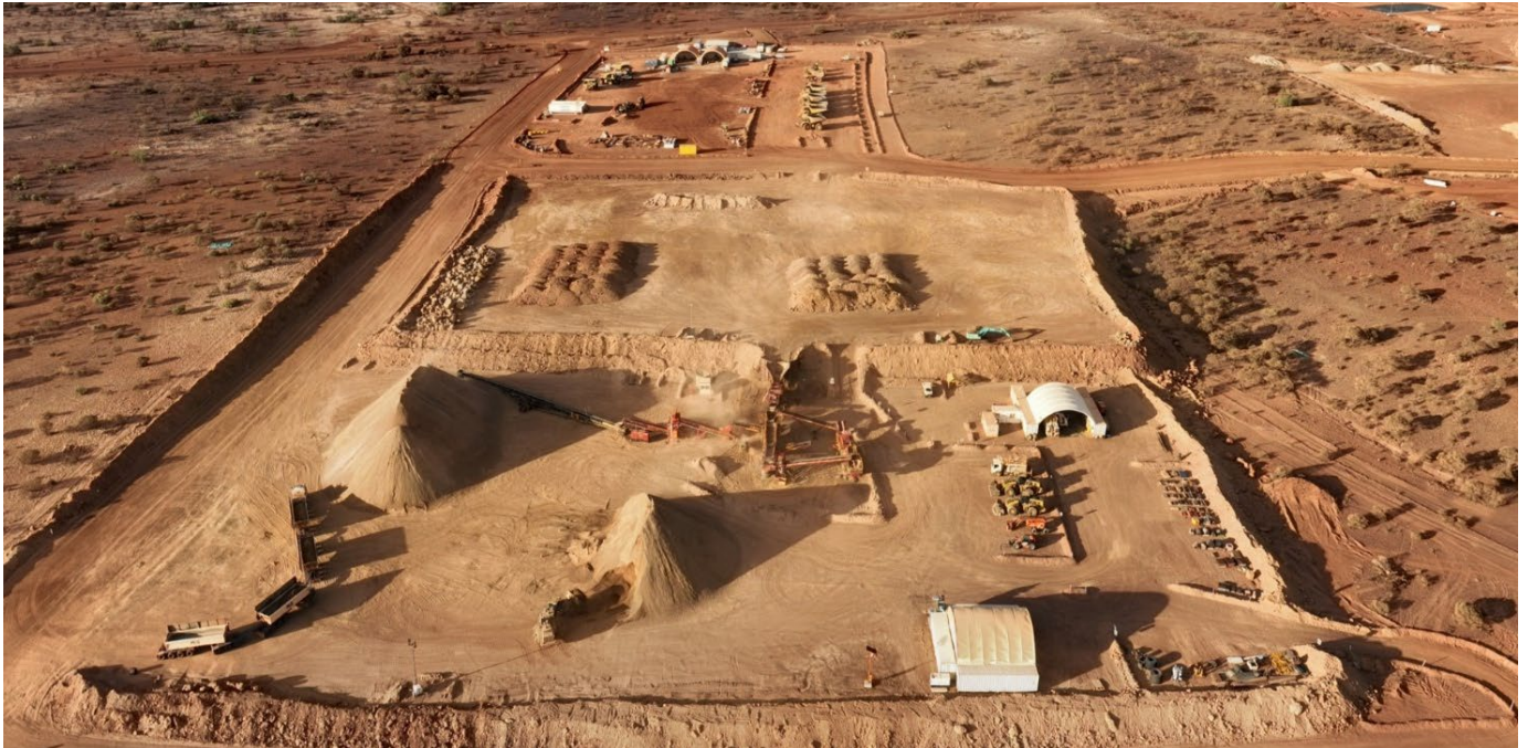
Figure 2: Crown Prince ROM and Crusher Pad
