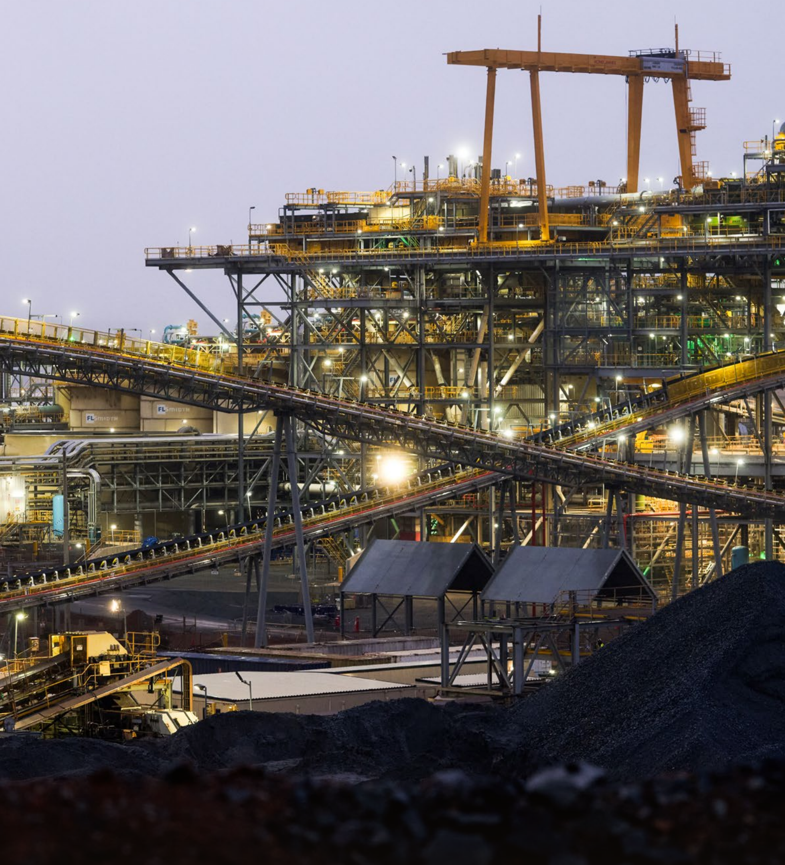
Processing Plant KCGM Operations Kalgoorlie Production Centre, Western Australia
