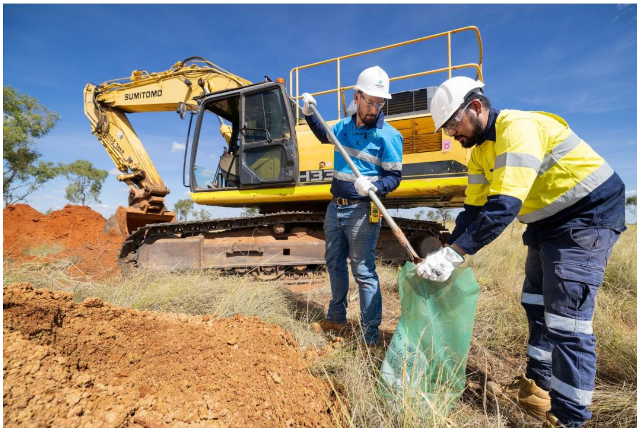
Figure 5 – Test pitting for input into engineering designs
