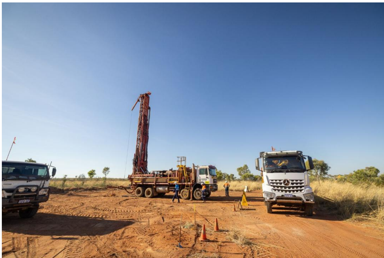
Figure 6 – Construction of water production bores
