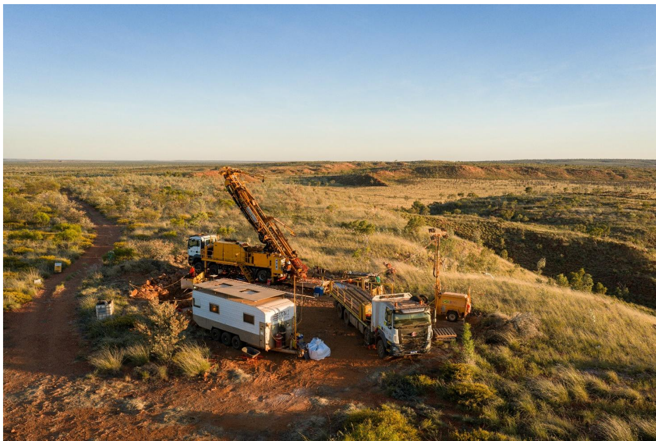
Figure 10 – Dazzler geotechnical drilling
