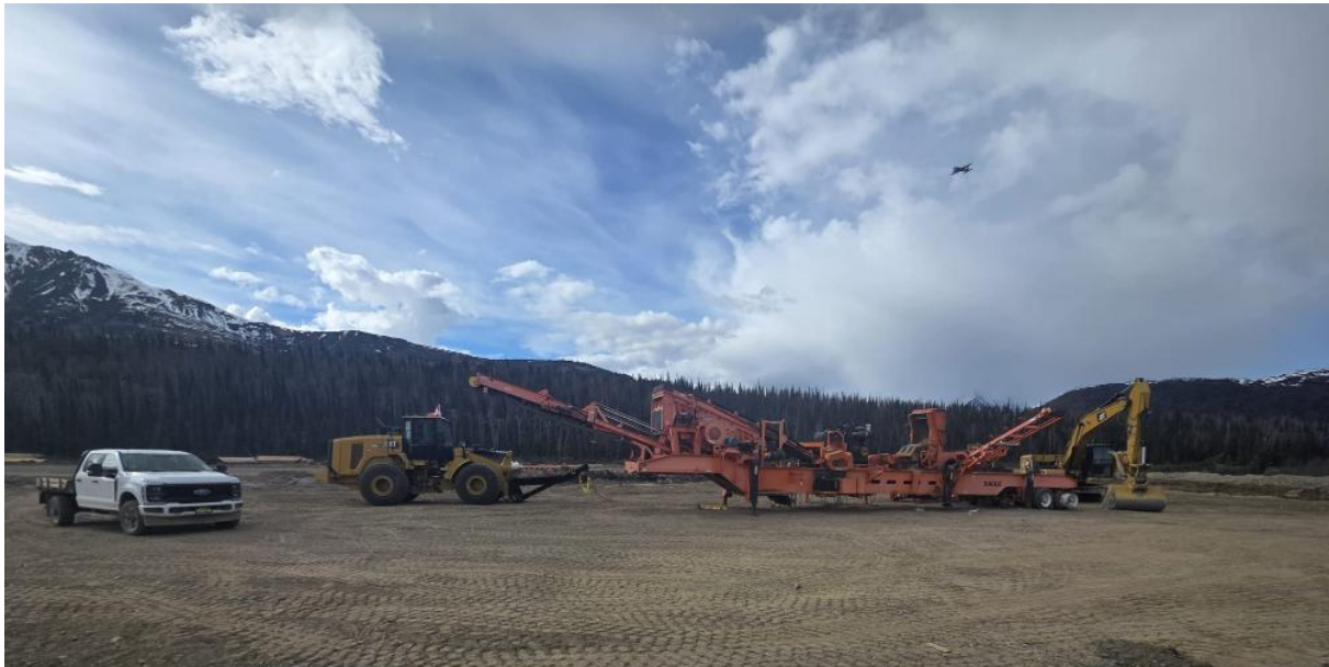
Figure 2. Crusher screener plant assembly in process at Whiskey Bravo site.
