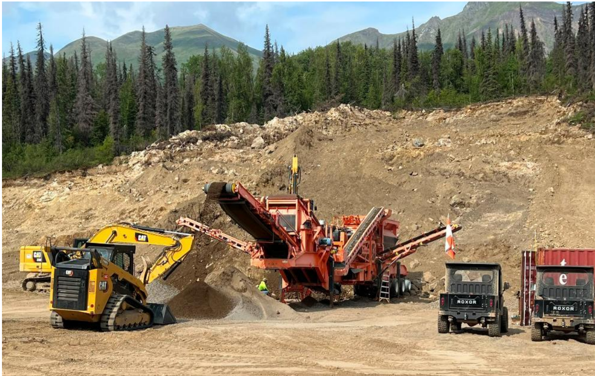
Figure 3. Gravel quarrying for the Stibium trail, airstrip expansion and ore sorter site
