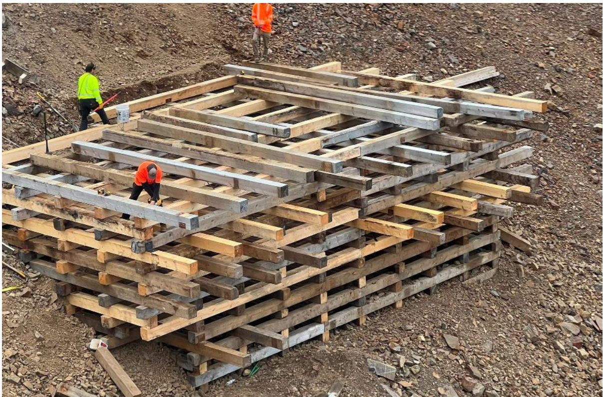
Figure 6. New pad being built at the bottom of the ridge at RPM
