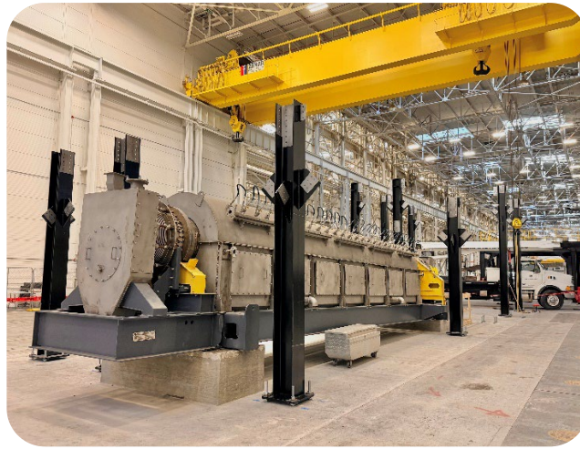
Figure 2 Agglomeration (Installation in Progress)
