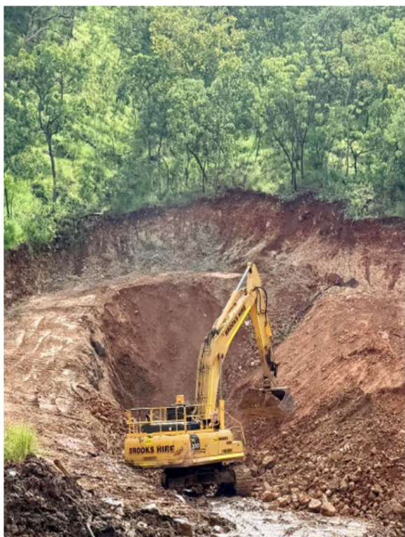
Plate 1 – Ground stability and box cut earth works
