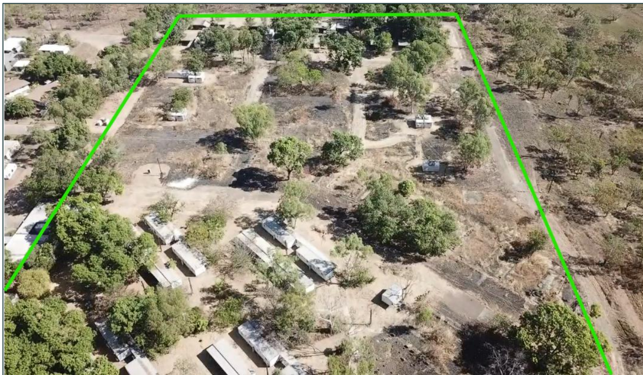
Figure 5. Drone imagery of Territory Iron Camp (looking west)
