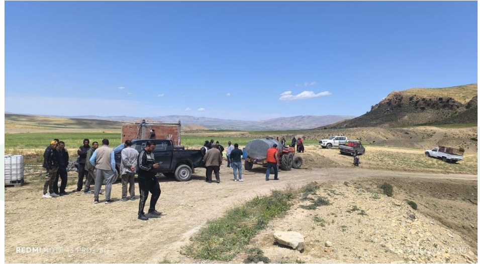
Repair of community water infrastructure by PhosCo
