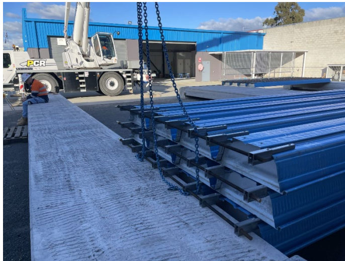
Image 3: SlimDek210 Module lifting arrangement
